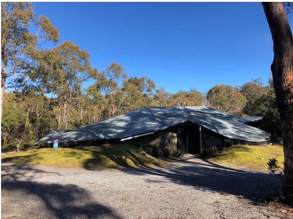
Figure 3 Central amenities building
