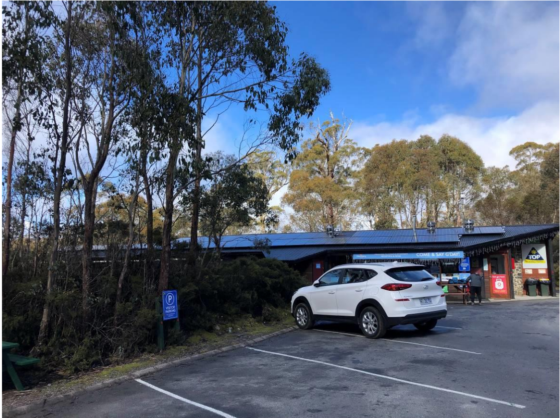
Figure 4 Existing reception building
