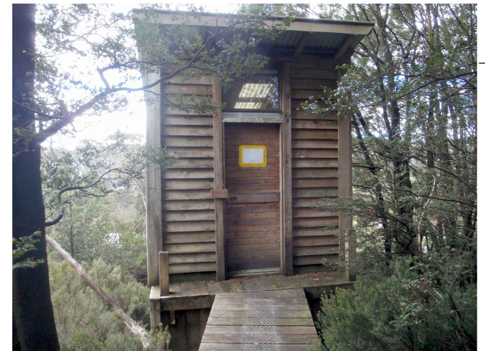
Image 5: Old toilet/store to be demolished
