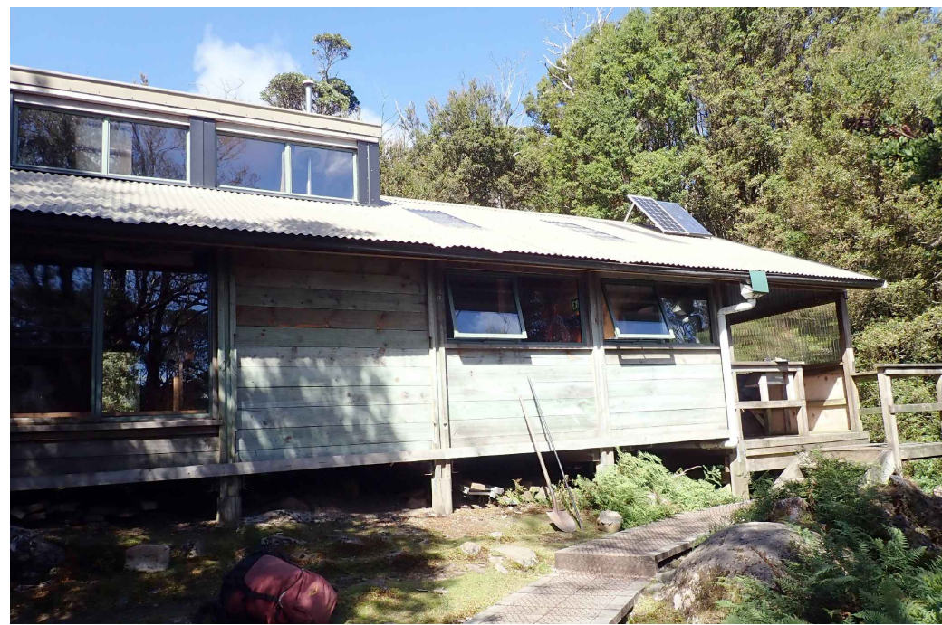
Image 2: Public hut RHS to be demolished
