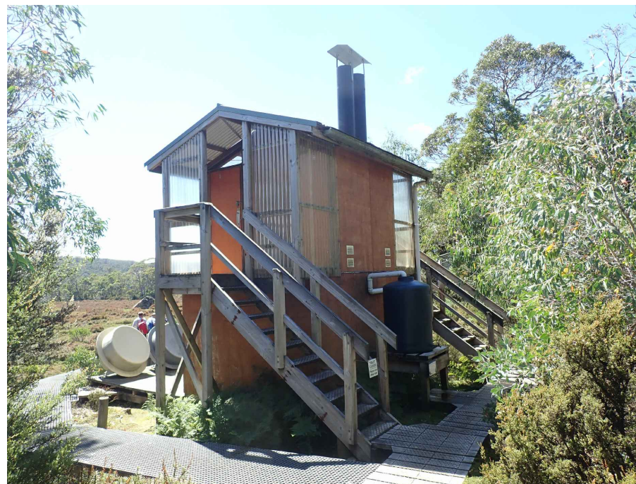
Image 4: Toilet to be demolished
