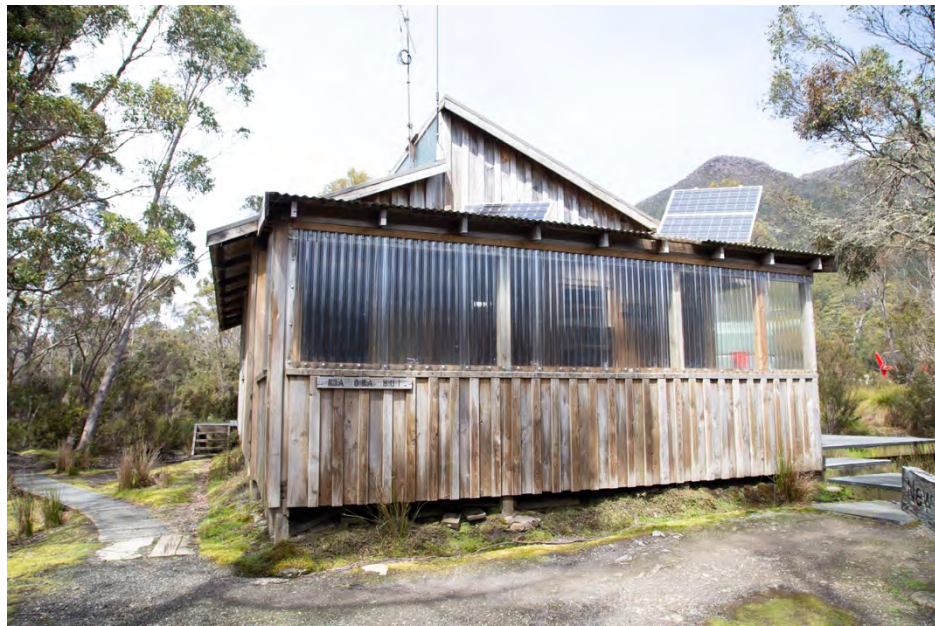
Photograph 2 Existing Kia Ora Hut
